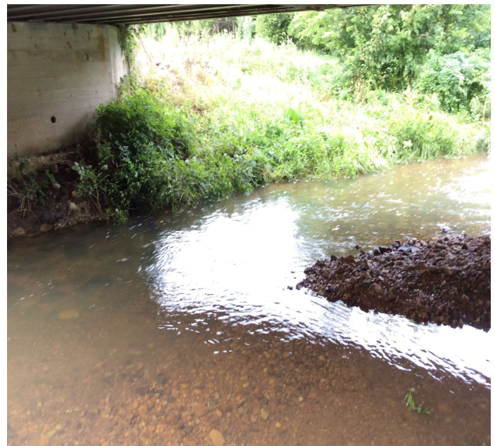
PHOTO 2 Description Channel has realigned towards Abutment 1.
