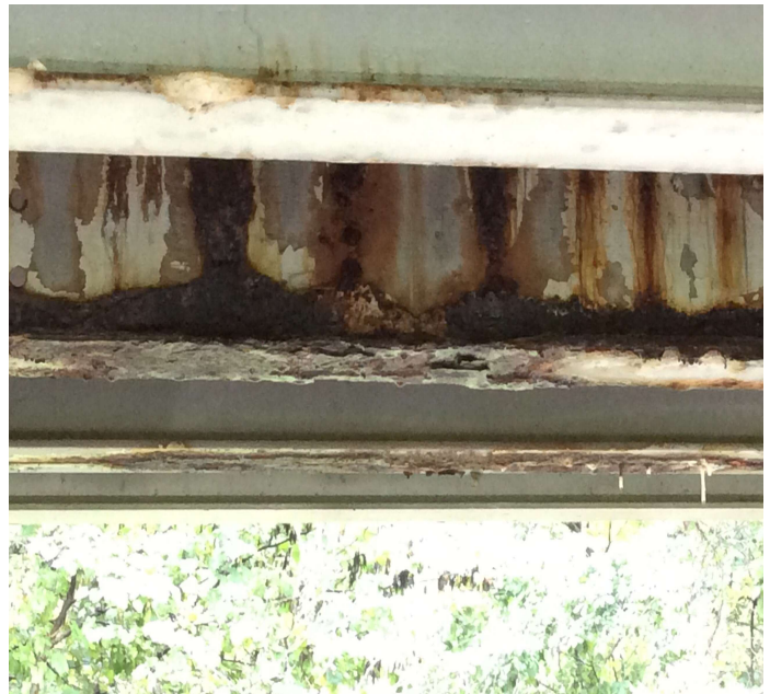
PHOTO 2 Description Girder 10 has areas of rust and section loss with knife edge to bottom flange.
