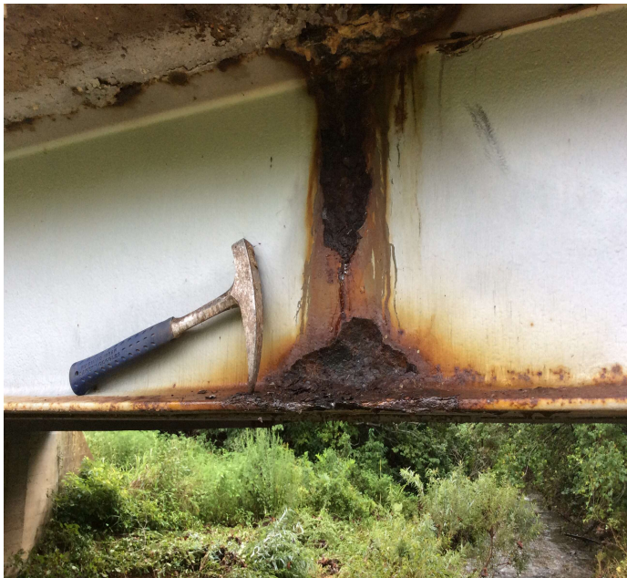
PHOTO 1 Description Girder 1. Areas of rust with heavy section loss to web & knife edge to bottom flange.
