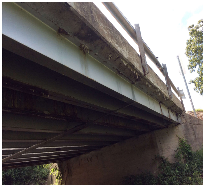
PHOTO 2 Description Left overhang efflorescent cracks.
