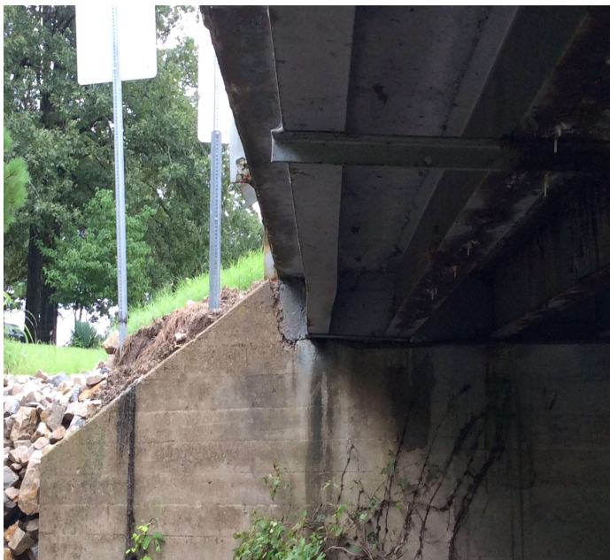
PHOTO 3 Description Girder 12 is bowed inward near Abutment 1.
