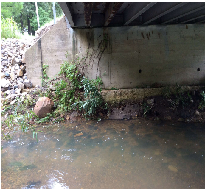
PHOTO 1 Description Channel is Scoured 3' below footing at Abutment 1 Right side.
