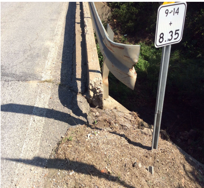
PHOTO 1 Description Bridge Rail First post on Right side is bent at Abutment 1.
